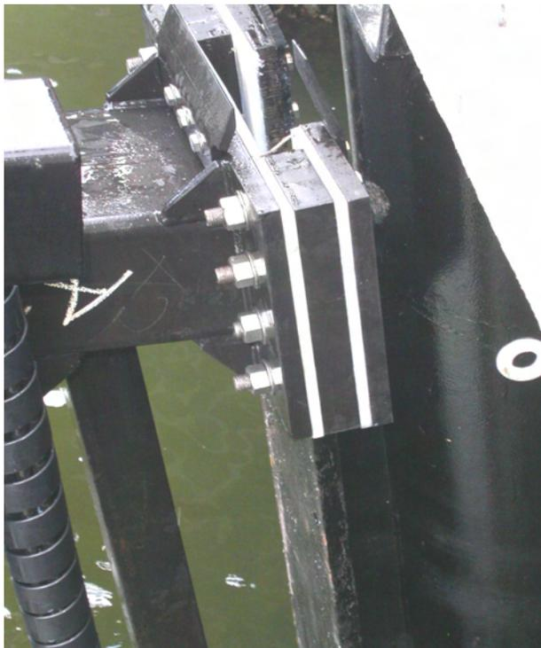
Figure 6: Mounting bracket
