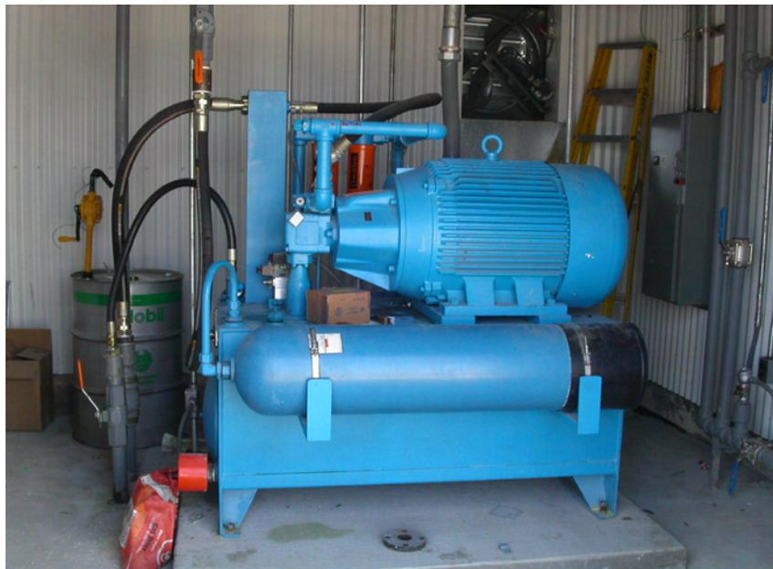
Figure 4: Hydraulic pumping unit
