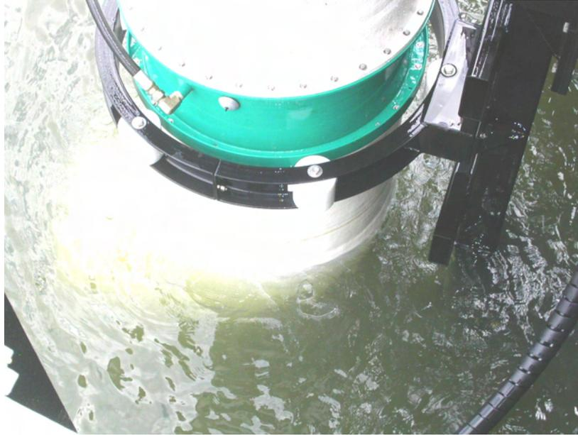
Figure 7: Jet attached to H pile
